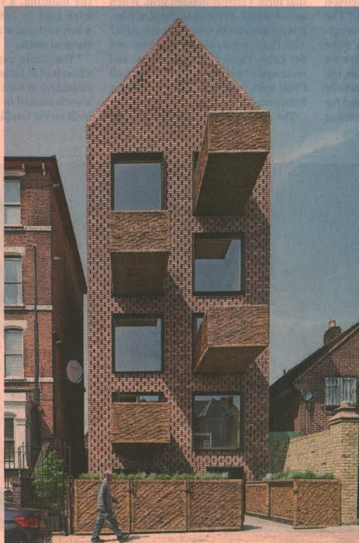
Barretts Grove's self-supporting brick façade and cantilevered wicker balconies Tim Soar
