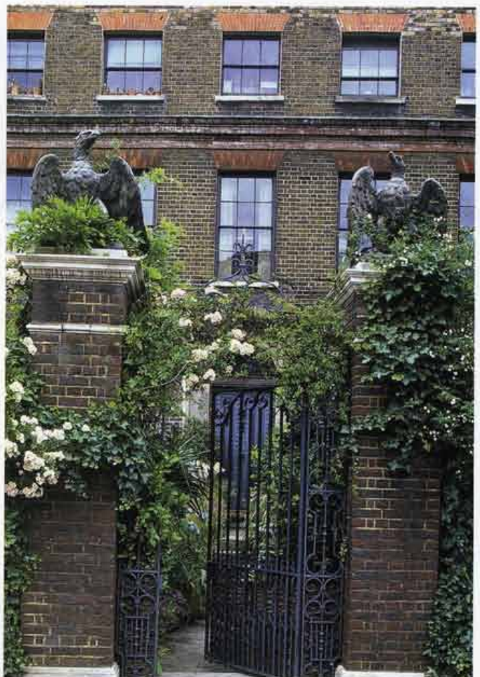
4—Restoring the frontage included making new front walls and ironwork. Rosa Kew Rambler cascades over the gate
